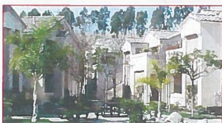
Arroyo Vista Apartments, Mission Viejo, CA 14 Units/Acre
